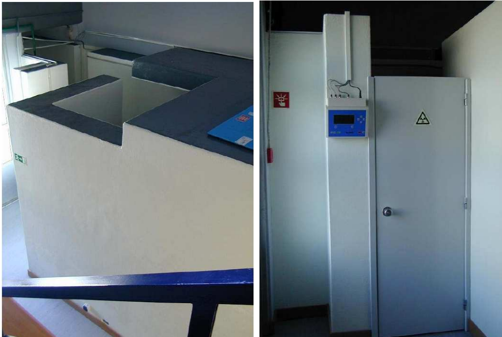
Figure 2.1: Top view of the hot lab with 30 cm thick concrete walls ( left ) and entrance to the bunker ( right ) where is visible the environmental radiation monitor.
