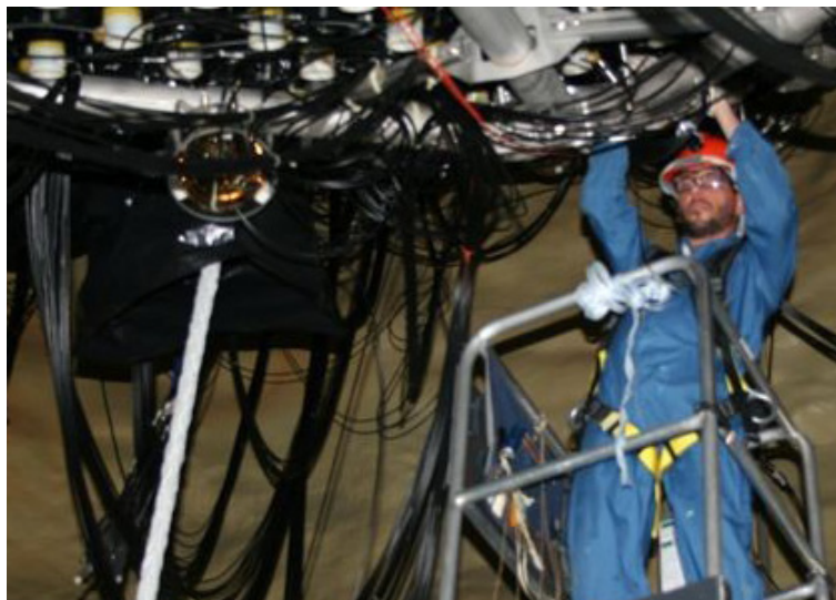
Installation of internal point of optical fibre in the PMT support structure.
